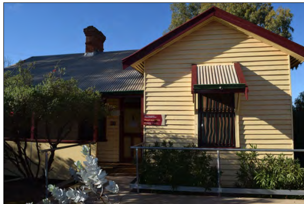
School Master's House, Goomalling.
