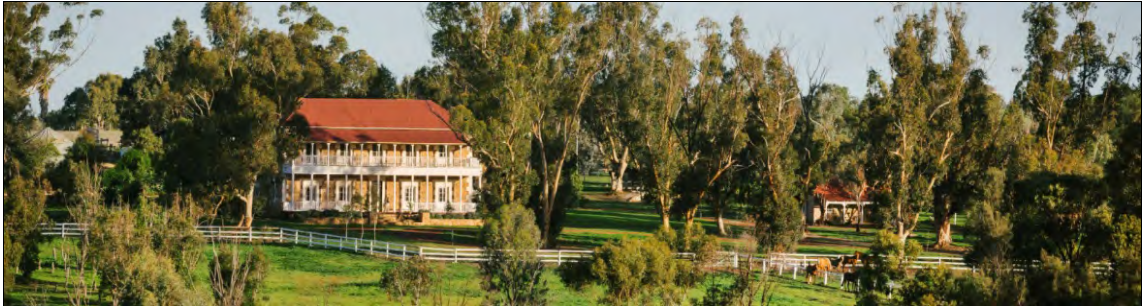
Buckland House and Property.
