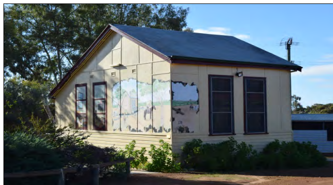
Refurbished Konogorrying School, Goomalling.
